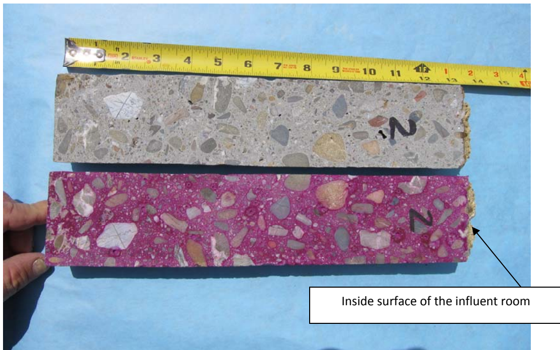
Photo 2) Macro-section prepared from roof slab core 2. The lower half of the core was stained with pH indicator (phenolphthalein). There is 13 inches of sound concrete in the roof slab at this location.
