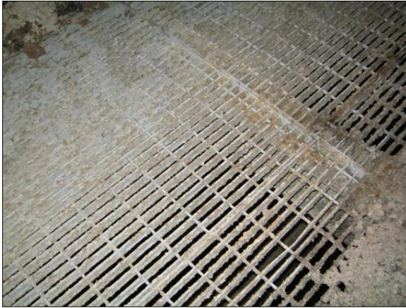
Photo 17. Aluminum grating in fair condition in most places.
