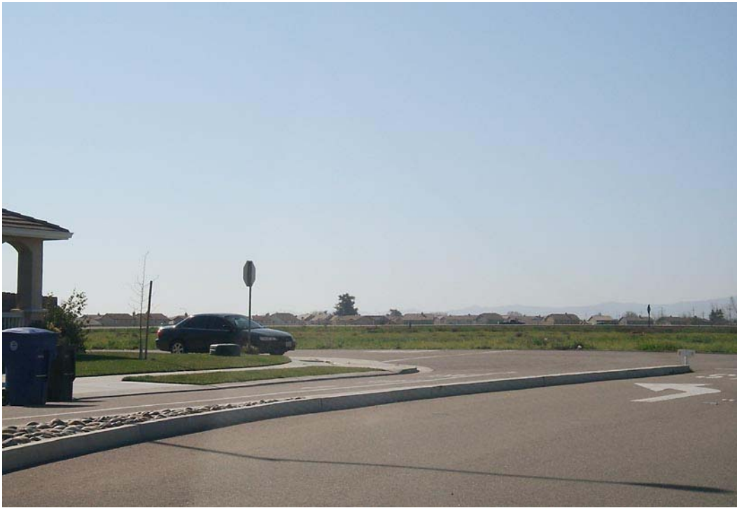
Viewpoint 7 – View of the project site looking south from Fishback Road. View of the middle portion of the project site is shown.
