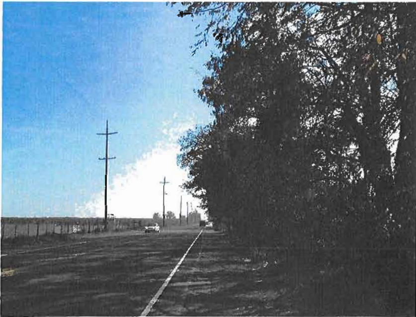
Photo 18 – East Side of Site
