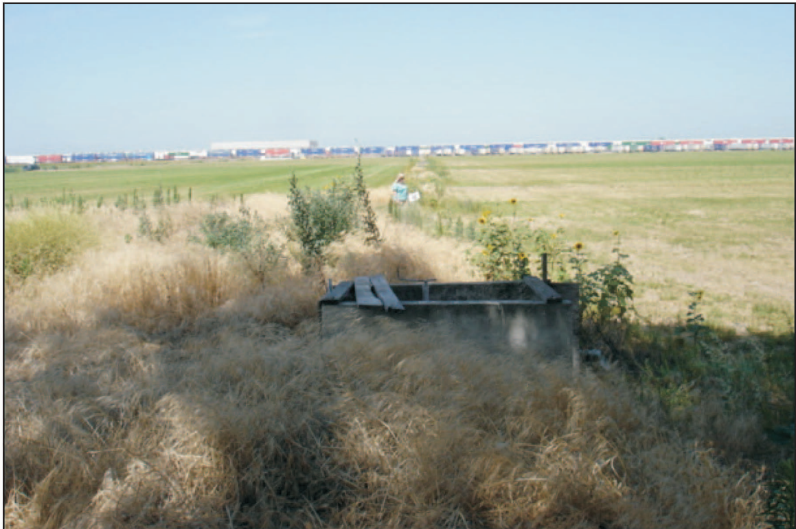
Photograph 4: Typical irrigation drainage ditch, facing west.
