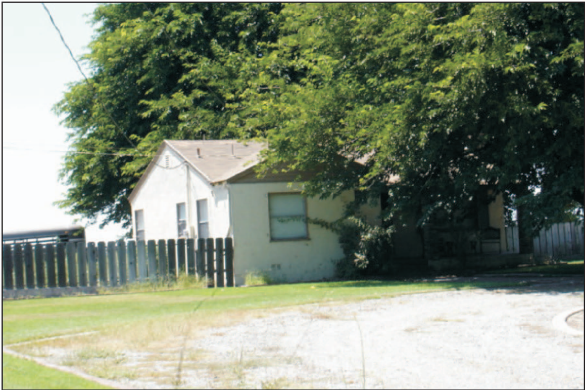
Photograph 9: Small residence at Aufdermaur farm, facing west.
