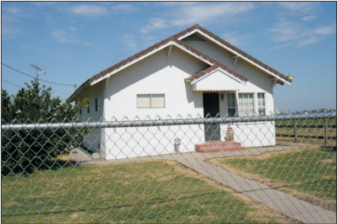
Photograph 5: Small residence along Airport Way, facing west.
