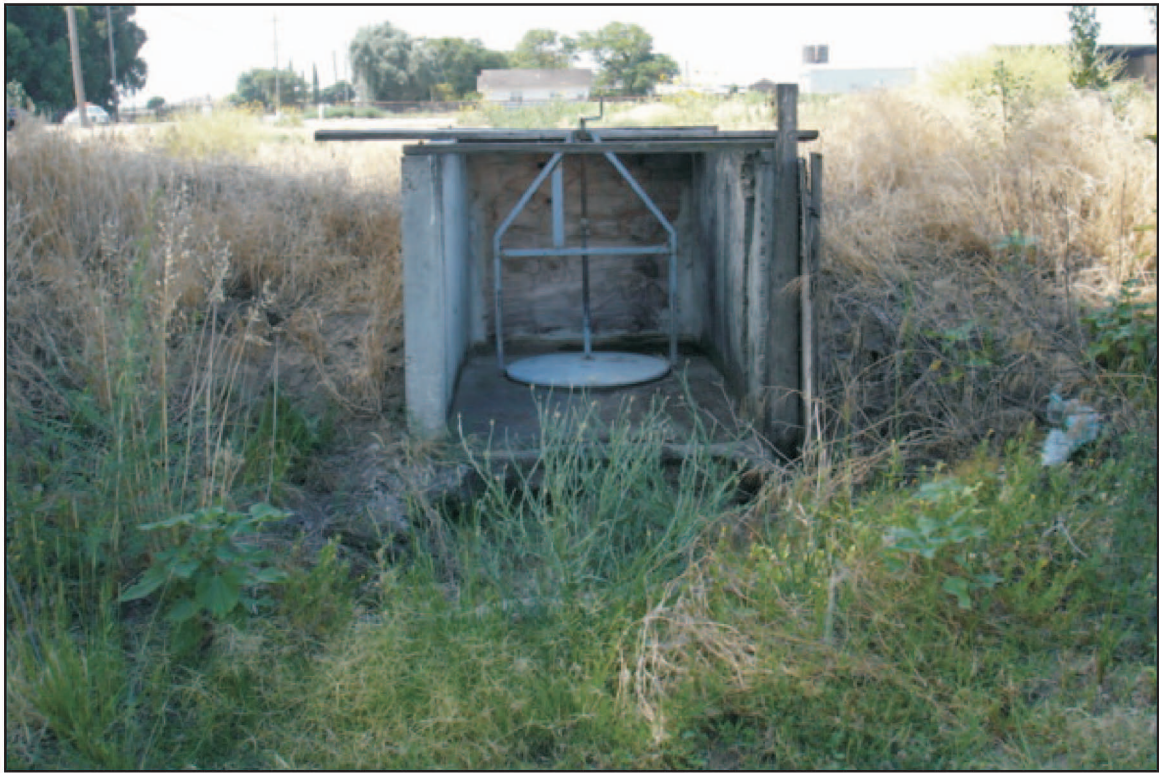
Photograph 3: Typical irrigation lock mechanism, facing south.
