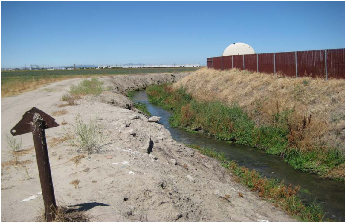
[2] DRAINAGE CANAL: (Facing west). Photograph was taken just west of the culvert (Photo 1) near the eastern property boundary. The Cal Suprema Cheese Factory is located within the fenced area on the far upper bank..
