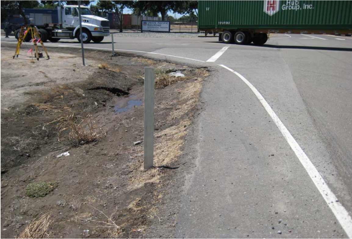
[9] ROADSIDE DITCH: (Facing West) Offsite portion of the roadside ditch as it veers south into the Union Pacific Facility. The drainage is shallow, with no continuous surface connectivity to downstream USACE jurisdictional resources, and lacks any discernable aquatic resources.
