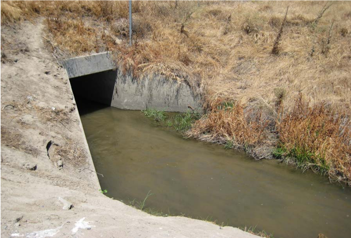
[5] DRAINAGE 1: (Facing northwest). Box culvert (Culvert 2) conveys flows from the Drainage Canal to the “French Camp Outlet” (See Photo 6) along the southwestern property boundary.
