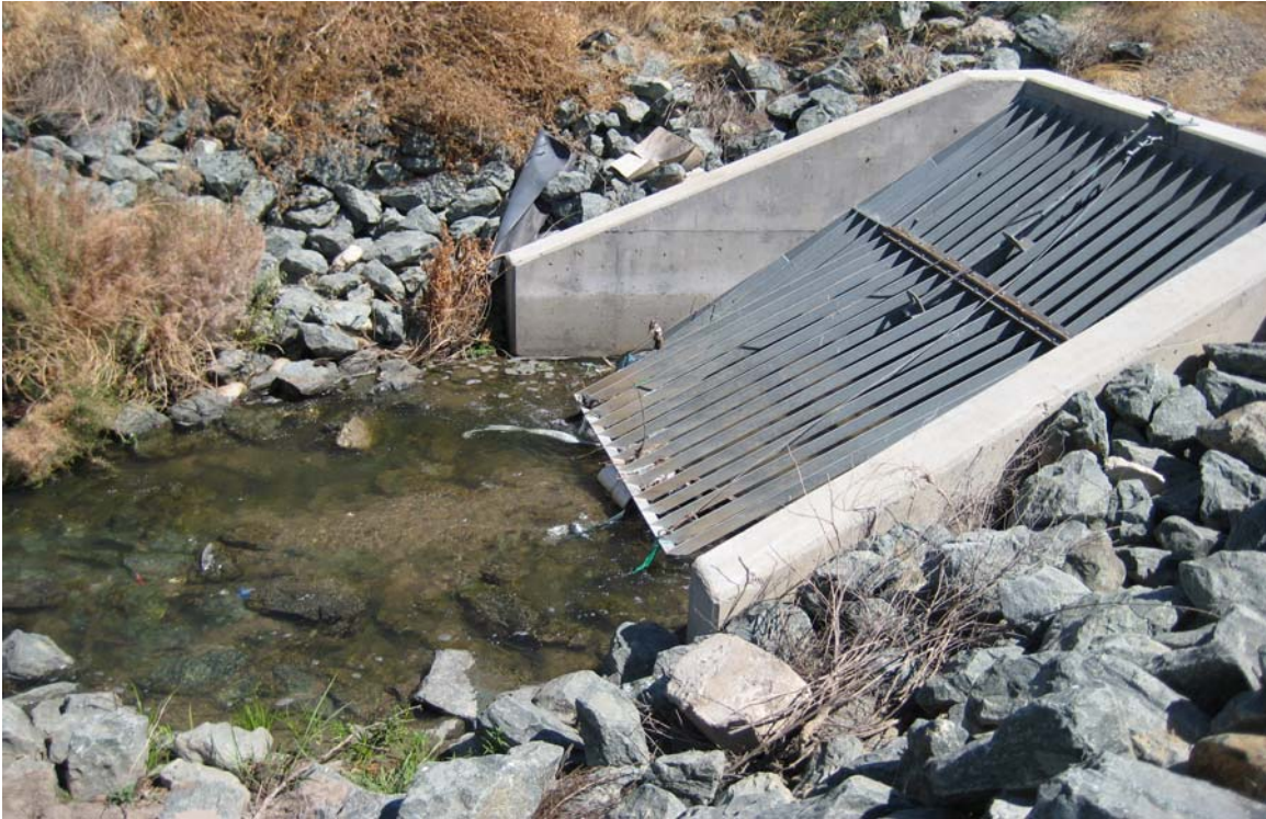
[1] DRAINAGE CANAL: Grated boxed culvert (Culvert 1) located near the eastern property boundary immediately south of the Cal Suprema Cheese Factory. The culvert conveys water from agricultural drainage ditches located east of S. Airport Way. Source water is diverted by the local irrigation district from the Stanislaus River located 10 miles to the south/southeast.
