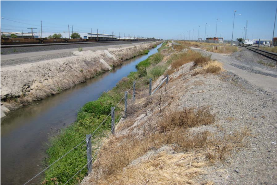
[6] FRENCH CAMP OUTLET: (Facing North). The off-site French Camp Outlet is the receiving water for the onsite Drainage Canal. The San Joaquin Sharpe Defense Depot is visible to the west (left) and the Union Pacific Lathrop Intermodal (Railroad) Terminal is visible to the east (right),
