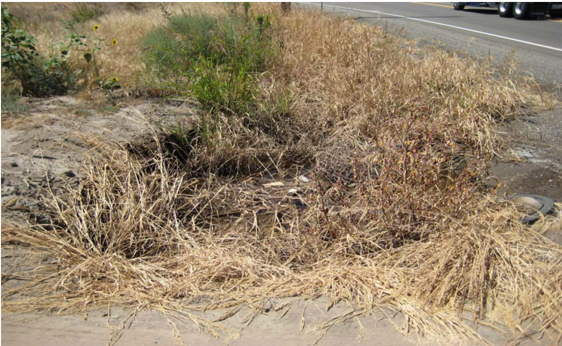
[8] ROADSIDE DITCH/CULVERT 3: (Facing West) A Small culvert is located at the northwest corner of the property. During the field visit, water was ponded near the culvert, originating from an undetermined source. Vegetation is dominated by upland species.
