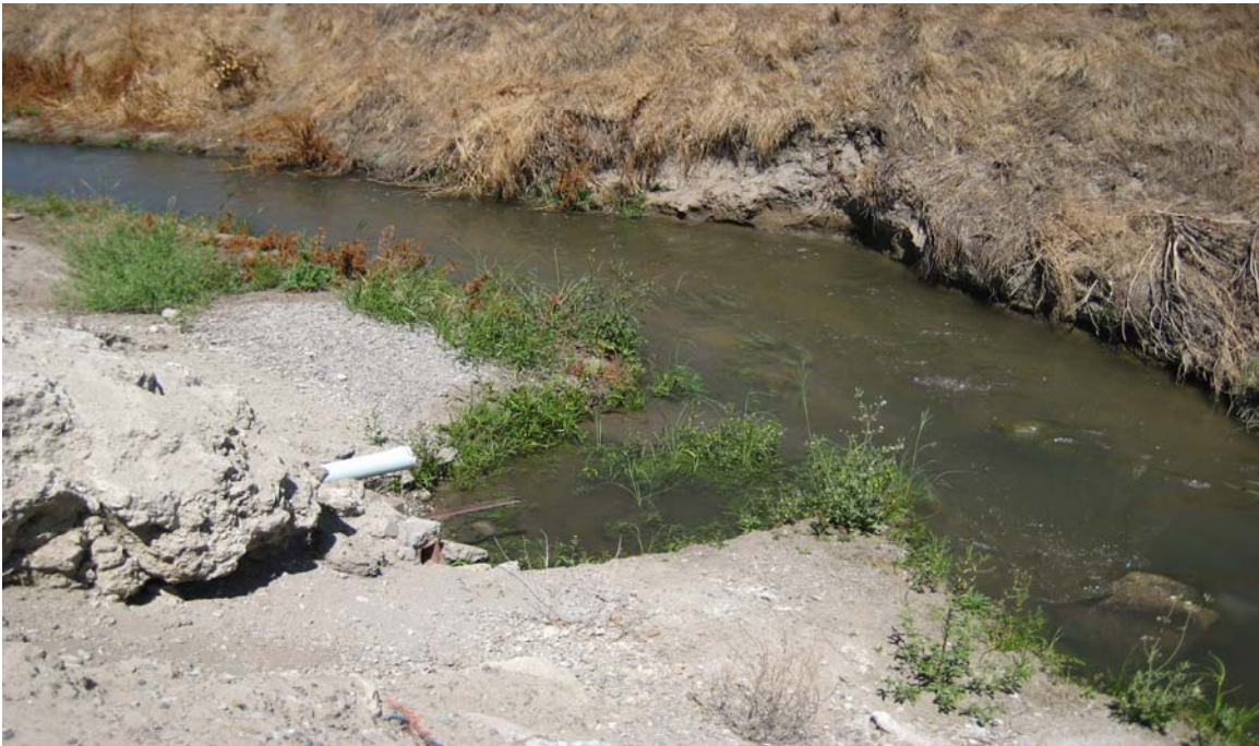
[4] DRAINAGE CANAL: Excess irrigation water from the adjacent fields to the south enter the canal through a network of PVC (3-4 inch) outlet pipes. No outlet pipes were visible on the north bank.
