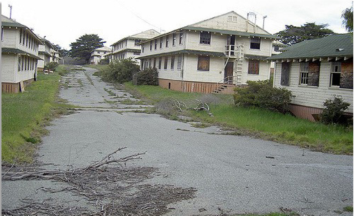
Much of the former Fort Ord property must be decontaminated before development can proceed.
