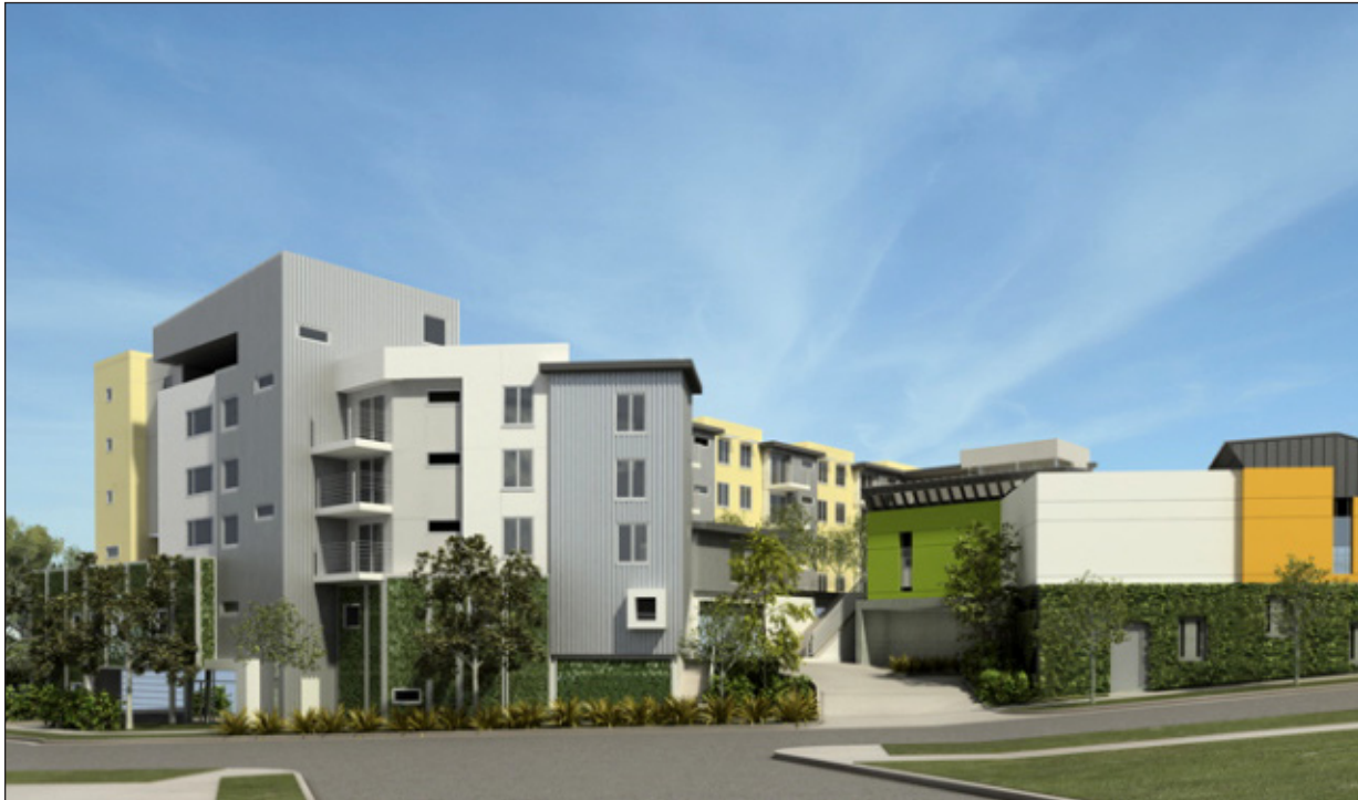
The northwest corner of the apartment block at Glassell Park.
