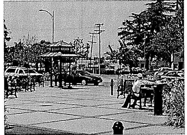
Plaza at Tidewater Bikeway and West Yosemite Avenue
