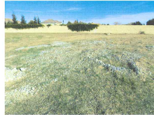
PHOTO 9: Gravel and concrete debris noted within southeast portion of the site.
