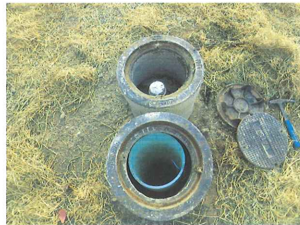
PHOTO 11: Utility vault boxes of electrical and water/sewer.
