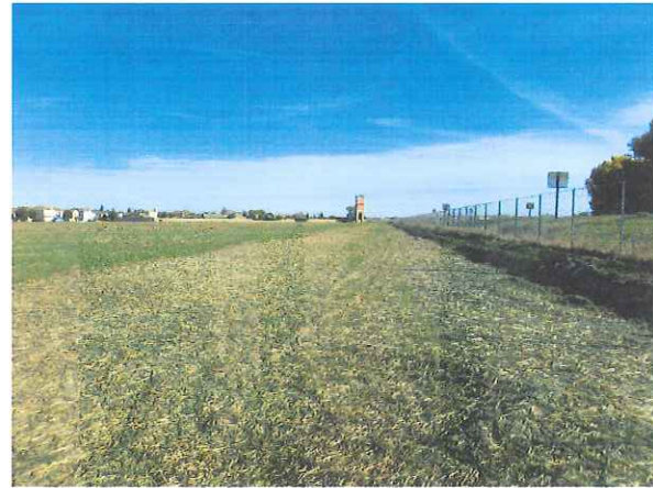
PHOTO 7: Looking east from southwest corner of site. Note low lying area and storm water pollution controls (seeding and straw).
