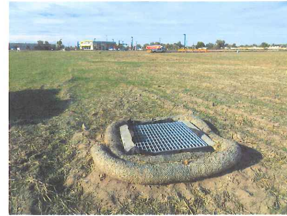
PHOTO 4: One of several utility drainage vaults noted at the site.
