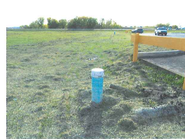
PHOTO 14: View of stubbed sanitary sewer casing along the site western boundary.
